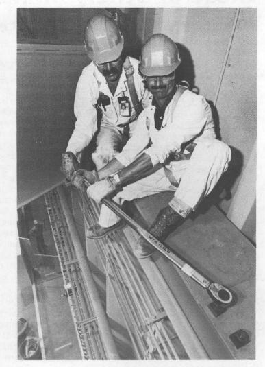
PRECARIOUS PERCH 30 feet above the floor — Sandia tradesmen Richard Parker (7814, left) and Mike Pacheco (7813) are harnessed to a high-bay bridge crane in Bldg. 820 as they tighten a fastener using a torque wrench. Richard and Mike are two members of the Operation Crane Rescue Project that worked on critically needed cranes and hoists during the last holiday break. Reggie Tibbetts, Supervisor of Crane, Hoist, and Rigging Team 7813-3, watches from below.
